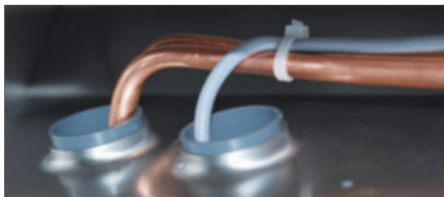
protective shrouds for cables and refrigerating lines
